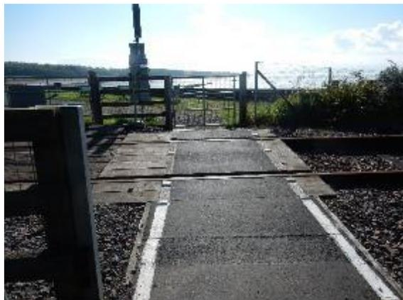
Low Valleyfield: OSGR NT006063 Restricted height and percussive surface over railway bridge. Ramped path provides alternative to steps on north side of railway.
