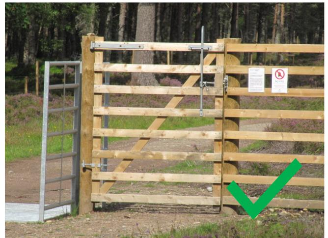
Where deer or livestock control is important, a suitable gate at least 1.5m wide should be installed adjacent or close to any cattle grid or locked gate. Make sure the ground under the gate and on the approach either side is level and firm.
