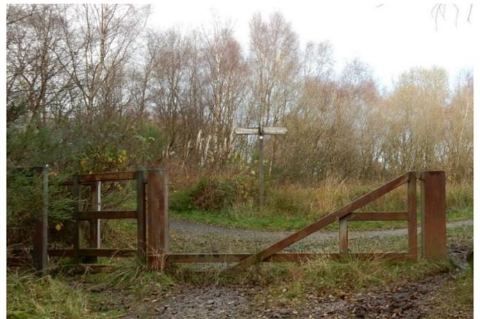
Elsewhere in Scotland, lockable vehicle barriers incorporating a horse stile have been used to good effect to restrict vehicular access whilst still maintaining equestrian access. The gap in the middle needs to be a minimum 1200 mm wide at the bottom and 2000 mm at the top. Timber rails over the lower section stop horses clanging their hooves on the metal.
