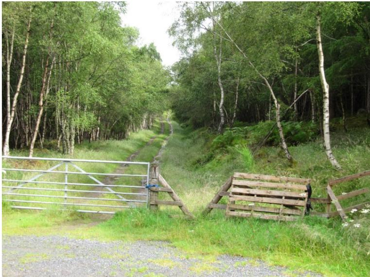
Informal wooden horse stiles such as this can easily be created but may be less effective at stopping determined motorcyclists than parallel sleepers or metal barriers
