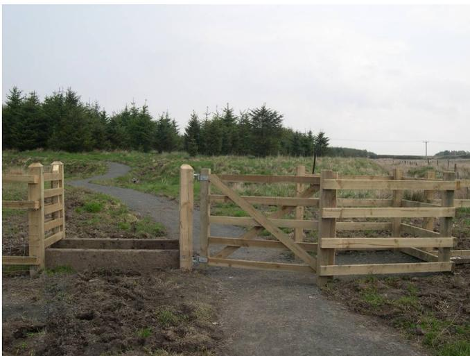
Provision of an adjacent kissing gate maintains unrestricted access for walkers. A RADAR gate would maintain access for wheelchairs too.
