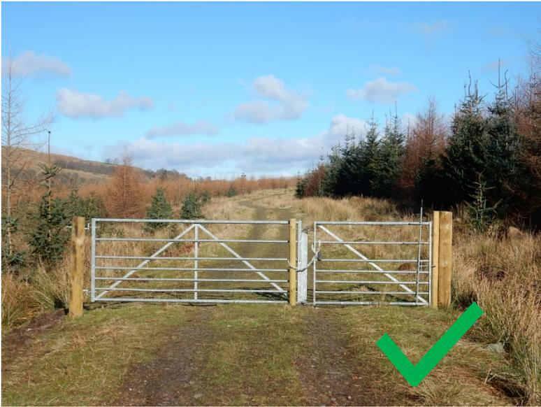
A side-gate minimum 1.5m wide adjacent to a locked gate, cattle grid or barrier will stop vehicles but still allow walkers, cyclists and horse riders access. Offset self-closing hinges will ensure the gate is stockproof. Commercially produced 1.5 m self-closing bridlegates with an integral H-frame are worth the investment to minimise future maintenance (available from [www.centrewire.com](http://www.centrewire.com) and [www.secureafield.co.uk](http://www.secureafield.co.uk))
