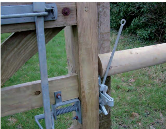
Following concern expressed by riders in the initial trial that the autolatch sticking out was a hazard, the extended stockproof handle and spring catch were removed and the extended handle autolatch also changed from the version commonly used in Devon (see above) to the version commonly used in Kent (see below), with a "D ring" on the gate instead of a prong.
